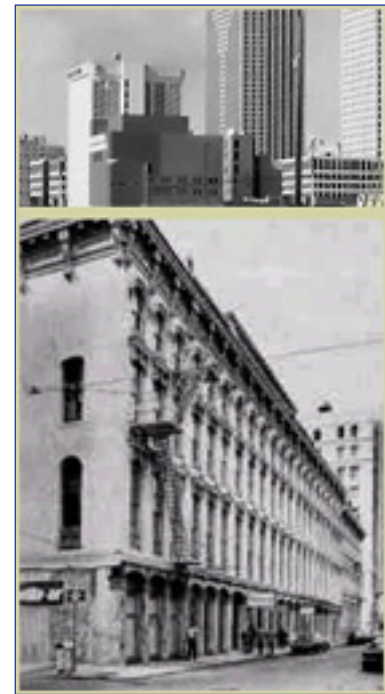
Fig 4: New Orleans' central business district is a blend of the old and the new. Both ultramodern skyscrapers and antebellum commercial row buildings can be found within its 14 square blocks.
